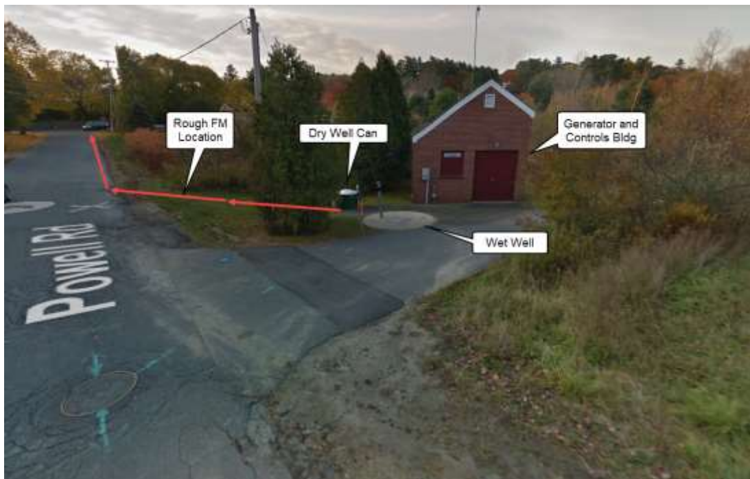
Figure 1: Powell Rd. Pump Station, Street View
