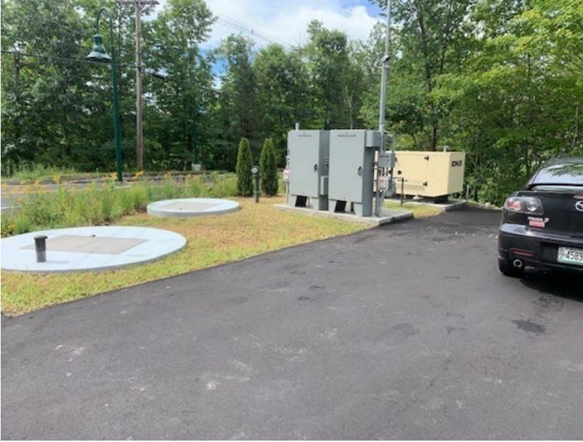
2019 CIP 180/3139, Phase 1 - new Depot Street Pump Station completed Fall of 2021
