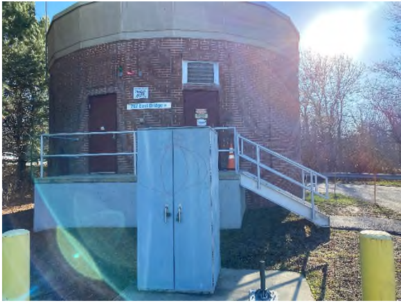
East Bridge Pump Station
