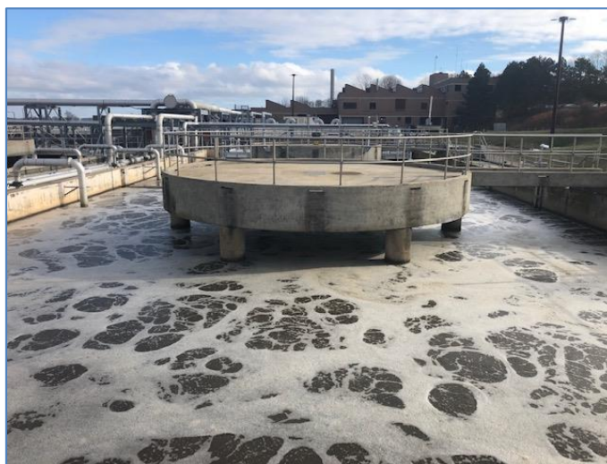
Aeration basin at East End Wastewater Treatment Facility
