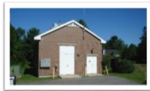
Continue to monitor chlorine booster stations in the distribution system to maintain WQ.
