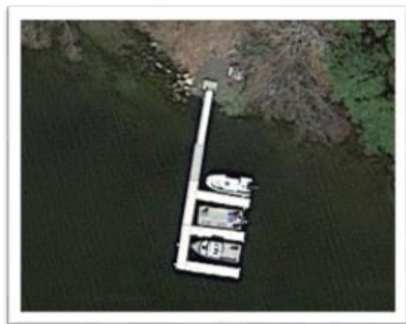
Secured the boat dock at the 52 Intake with additional mooring blocks.
