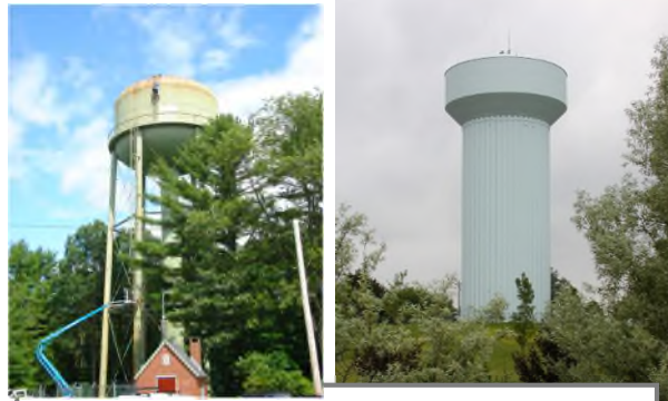
2019 – Subprogram 307 Elevated Storage for 407 zone north. This project will replace an old undersized 1950 Tank (left) with new tank (right) Currently under design – Construction 2021
