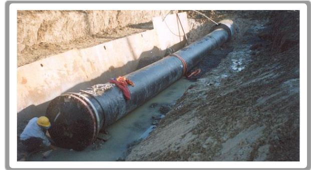
Design and construction support of Maine Turnpike infrastructure crossings
