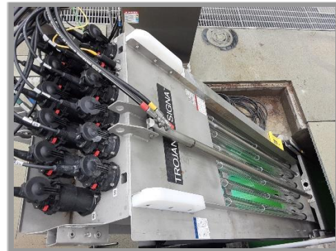
Managed CEWWTF UV Disinfection construction
