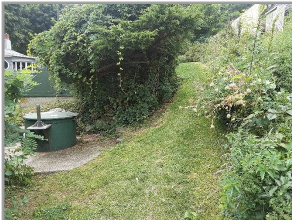
Manage design and construction of Maiden Cove Pump Station upgrade project.
