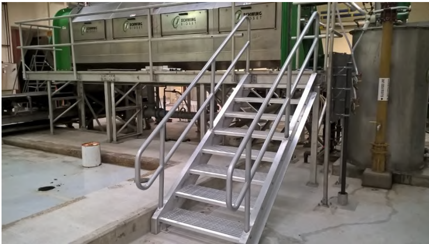
2018 CIP 416 project 3027 - Screw Press Access Stair and Platform
