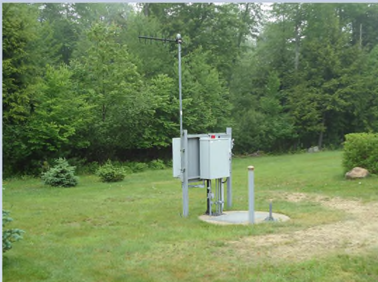
Park South – condition rating is 3.2 out of 5
