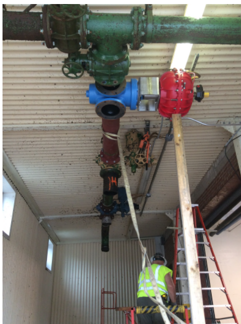
2019 CIP 416 project 3001 - Cake Unloading Valve during installation
