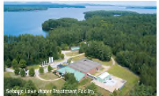
Sebago Lake Water Treatment Facility
