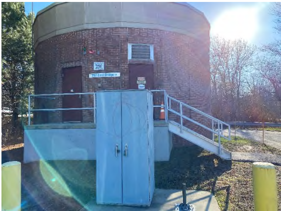
East Bridge Pump Station
