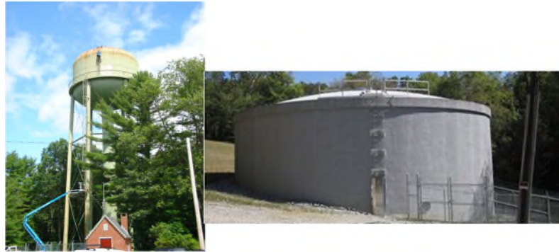
2019 – Subprogram 307, project #3004 Water Storage for 407 zone north. The project will replace an old undersized 1958 Elevated Tank (left) with new ground storage tank (right). Currently under design – Construction to start 2023 with anticipated completion summer of 2024
