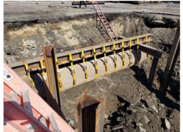
Pictured: India Street 33” pre-stressed Force Main exposed during installation of City Storm Sewer in 2019
