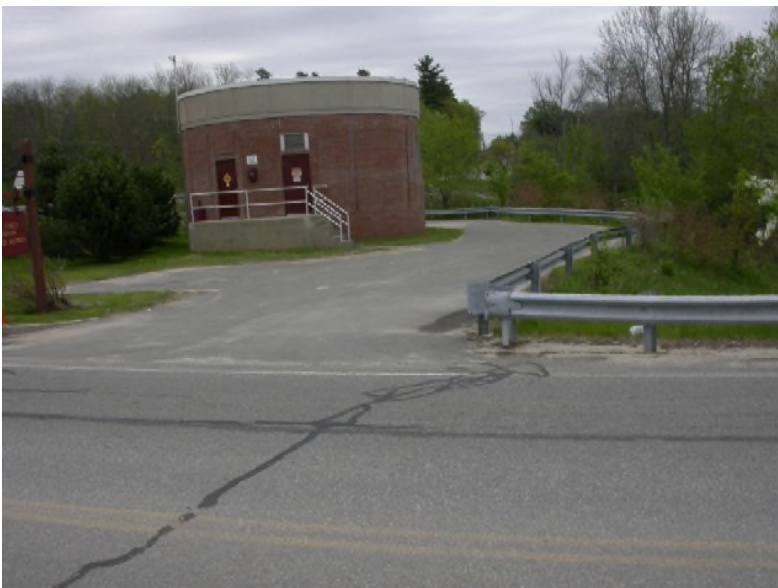
East Bridge PS roof replacement completed fall of 2023
