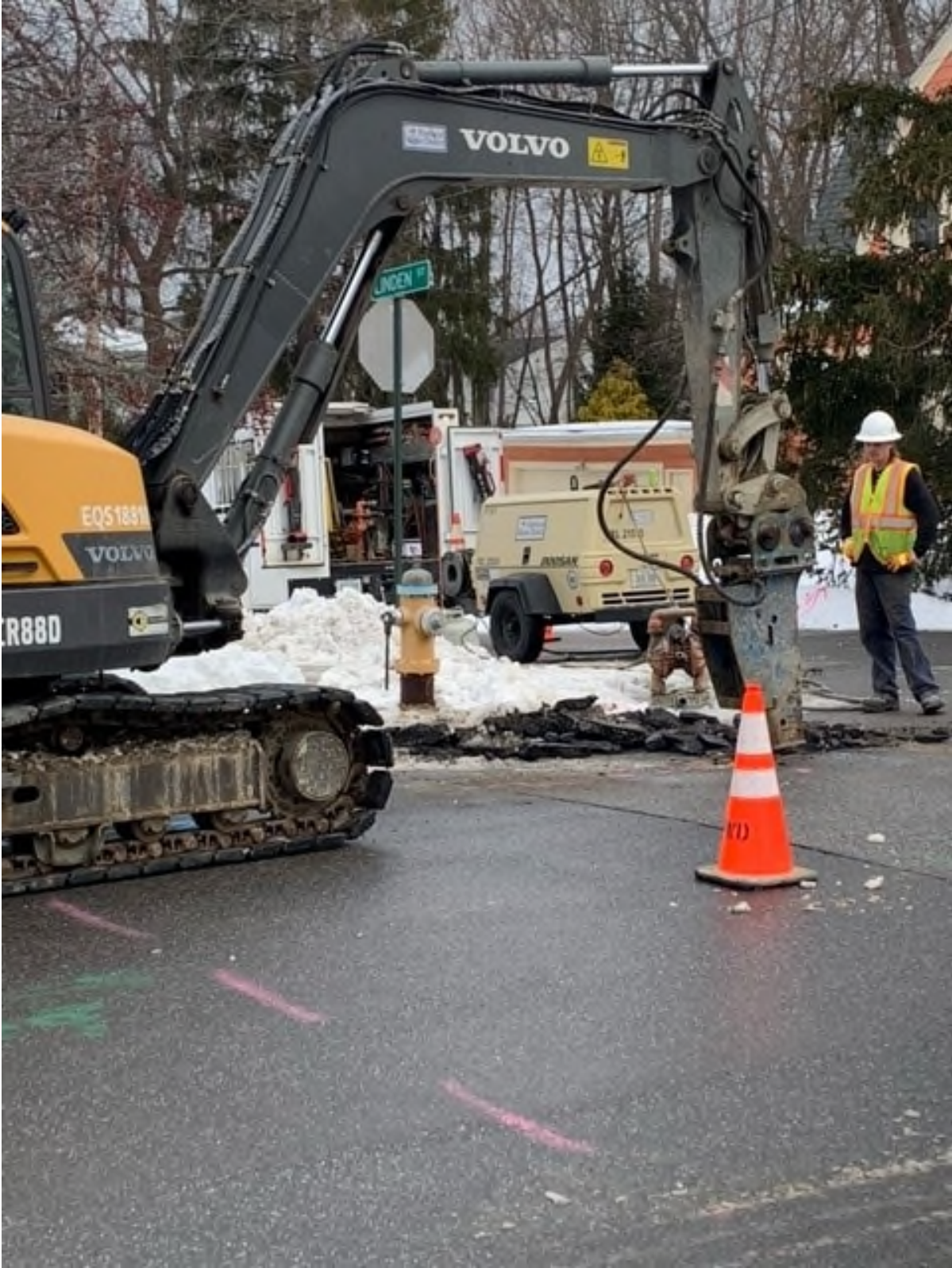
Crews repairing water main break on February 2, 2022
