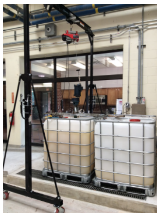
2019 CIP 416 project 3026 - Polymer System Improvements
