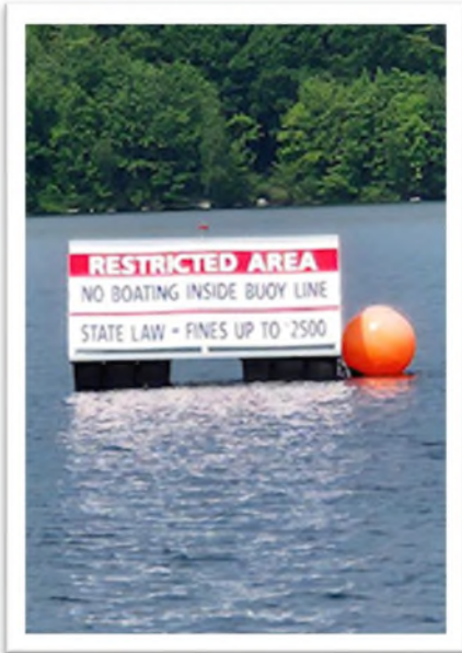
Redesigned the floating sign platform at the apex of the 3,000’ No Trespassing zone. This redesign proved to be more stable in rough, storm-driven waves.
