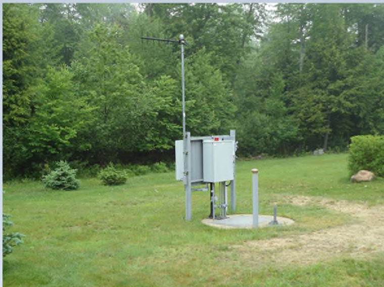
Park South – condition rating is 3.2 out of 5
