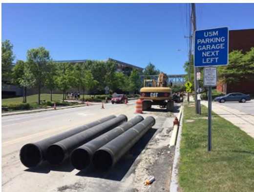
2019 CIP #43, Water Main Replacement project – Bedford Street, Portland
