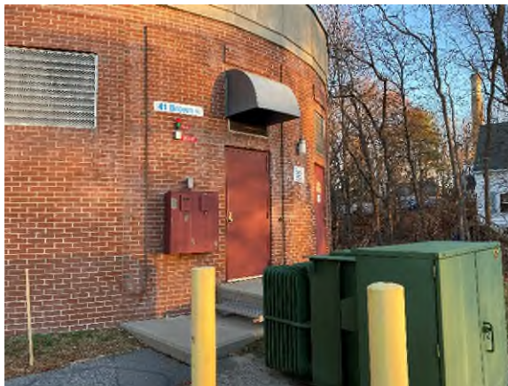
Cottage Street Pump Station
