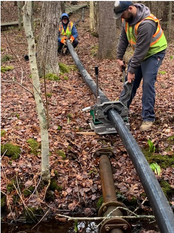
Fusing new 6" HDPE seasonal main
