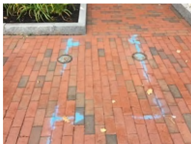
Locates for an 8" Fire Service and 4" domestic Service
