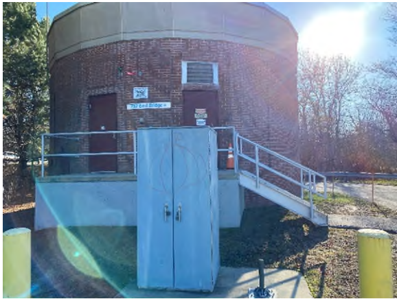
East Bridge Pump Station
