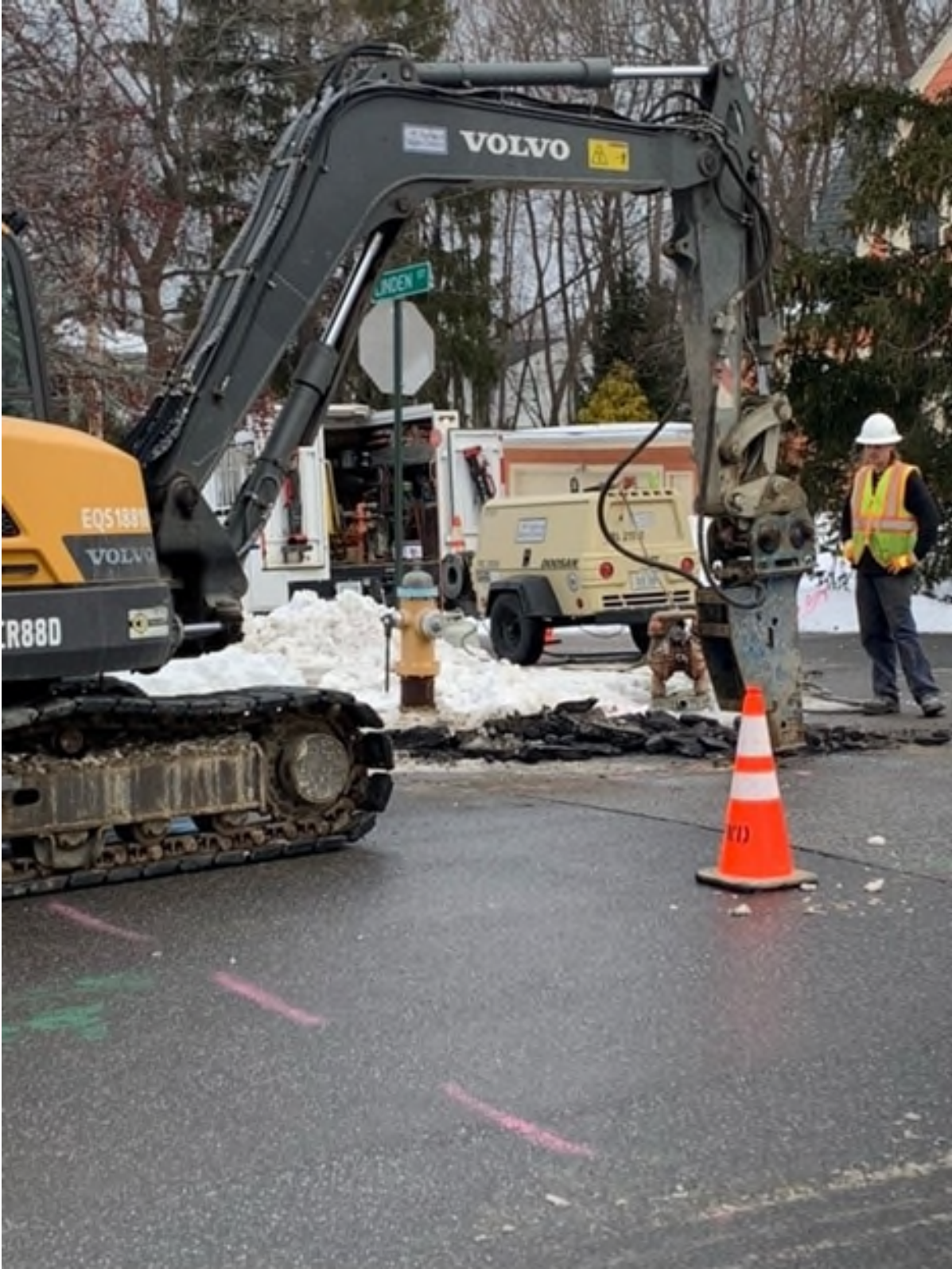
Crews repairing water main break on February 2, 2022
