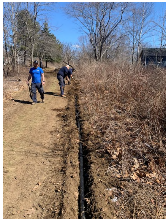
Chushing Island New 2" HDPE installed
