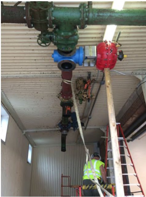
2019 CIP 416 project 3001 - Cake Unloading Valve during installation
