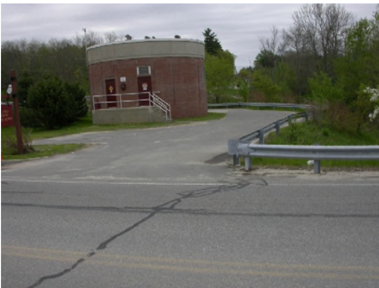
East Bridge PS roof replacement scheduled for 2023
