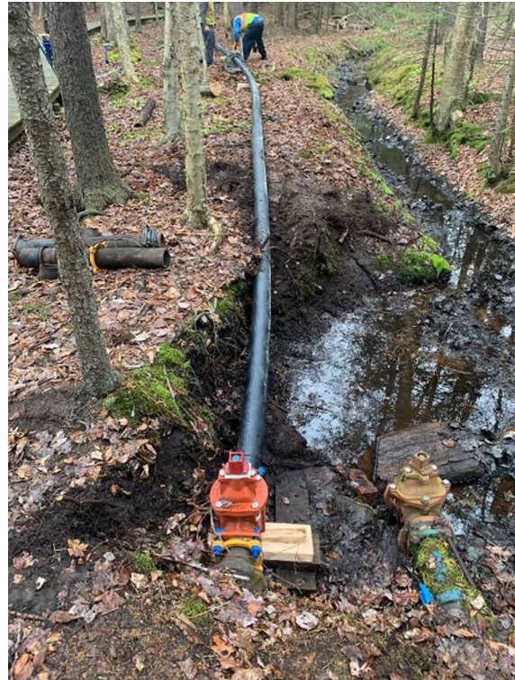
Sanctuary Ln., ROW Scarborough (boardwalk)
