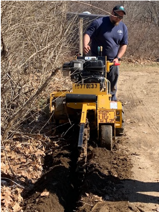
Chushing Island – Trenching for new HDPE
