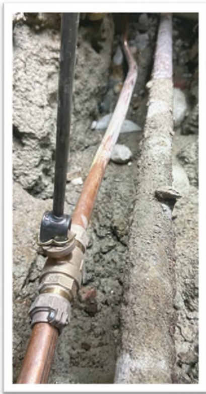
Replaced the last known lead service line in Portland, pictured to the right, with a new copper pipe, pictured to the left.
