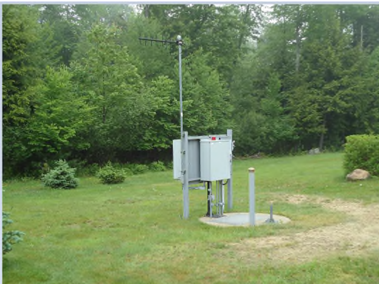
Park South – condition rating is 3.2 out of 5
