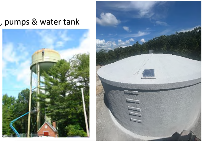
2019 – Subprogram 307, project #3004 Water Storage for 407 zone north. The project replaced an old undersized 1958 Elevated Tank (left) with new ground storage tank (right). Currently nearly completed with anticipated completion fall of 2024
