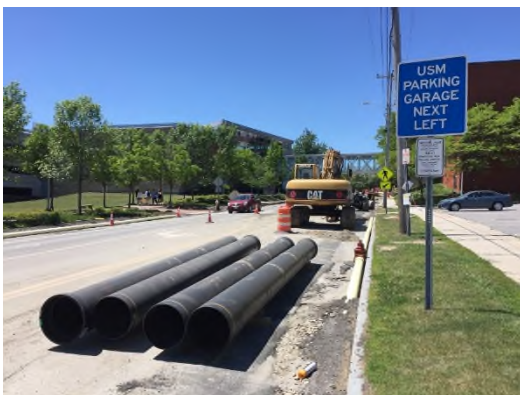
2019 CIP #43, Water Main Replacement project – Bedford Street, Portland
