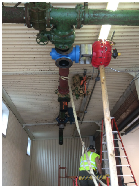
2019 CIP 416 project 3001 - Cake Unloading Valve during installation
