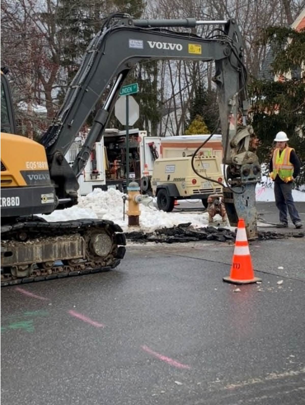
Crews repairing water main break in Portland
