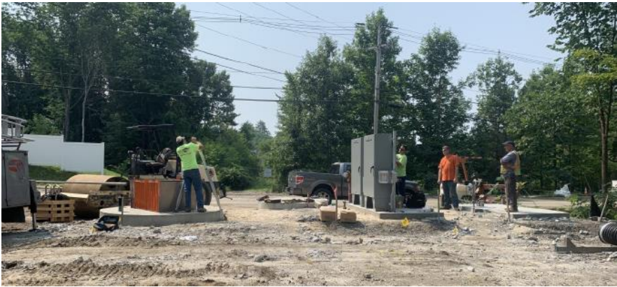
Contractor installing the Pump Station at Depot Street
