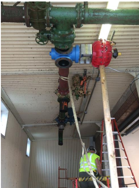
2019 CIP 416 project 3001 - Cake Unloading Valve during installation
