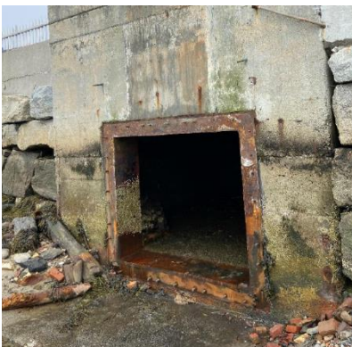
2019 CIP 131 -Tide Gate Replacement, India St. and Northeast Pump Stations: Currently under construction, completed summer of 2021.
