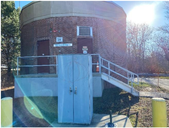
East Bridge Pump Station
